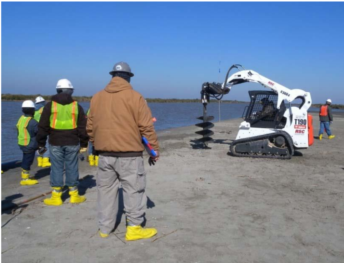
Figure 4.4 Pit Excavation Using Power Auger
