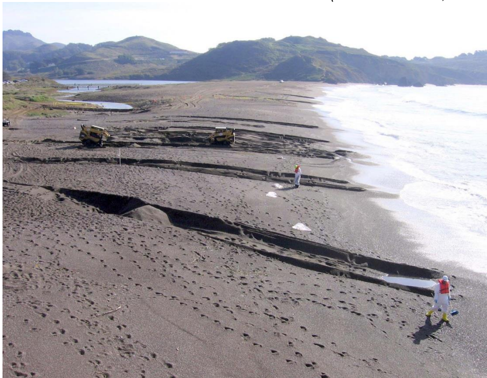
Figure 4.6 Mechanically-excavated Pit, and Across-beach Trenches Using Track Hoe
